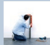
1. Align the back profile and fix it (screw it) to the wall
